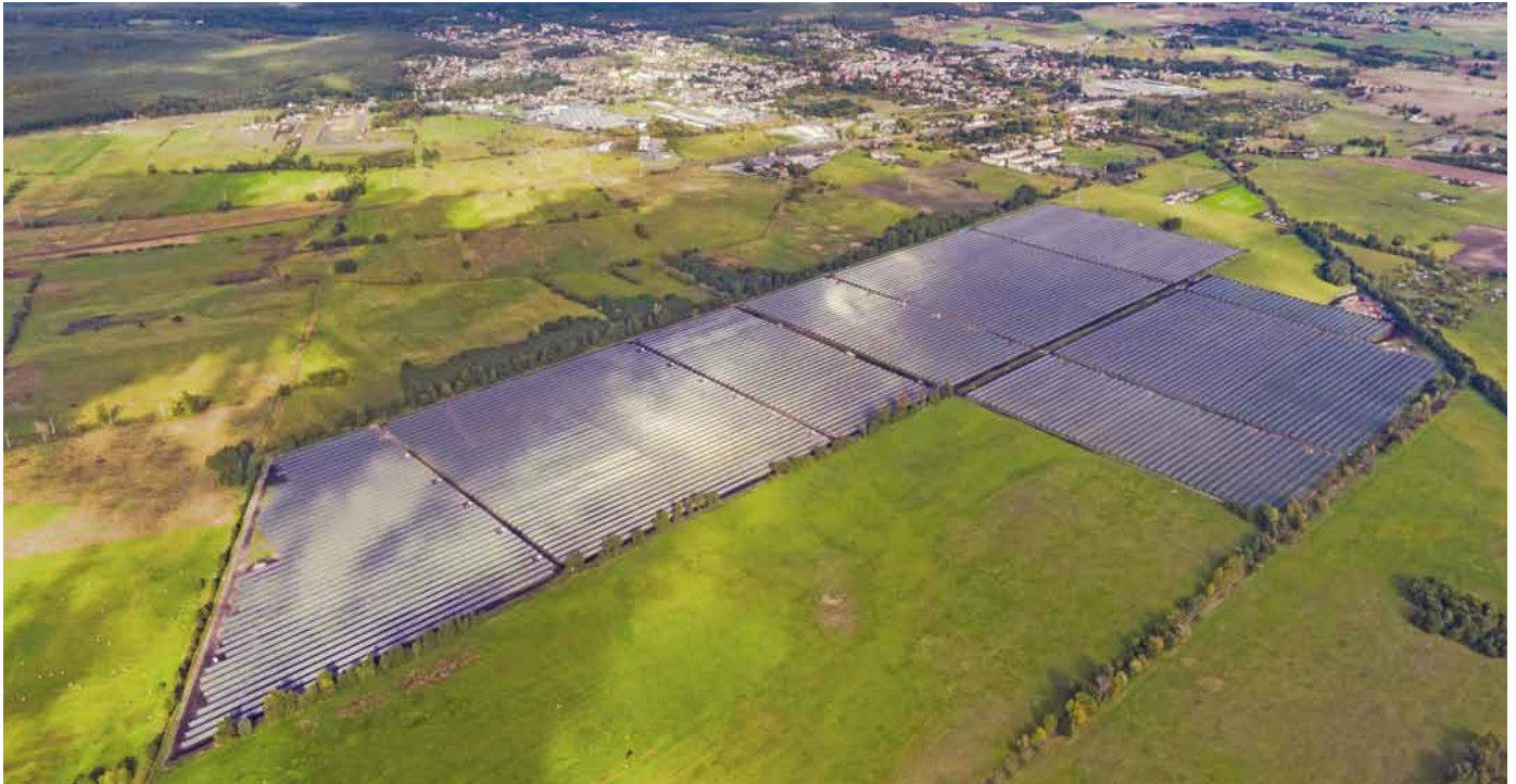
The 65 MW Witnica Solar Farm in western Poland is set for completion in the first half of this year, and will power a nearby cement factory under a 10-year private power purchase agreement.
